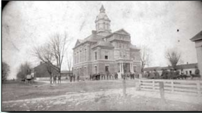
The Old Boone County Courthouse was built in 1889, but the County has never had a set of plans for the building until last summer when UC students completed a set of detailed drawings.
